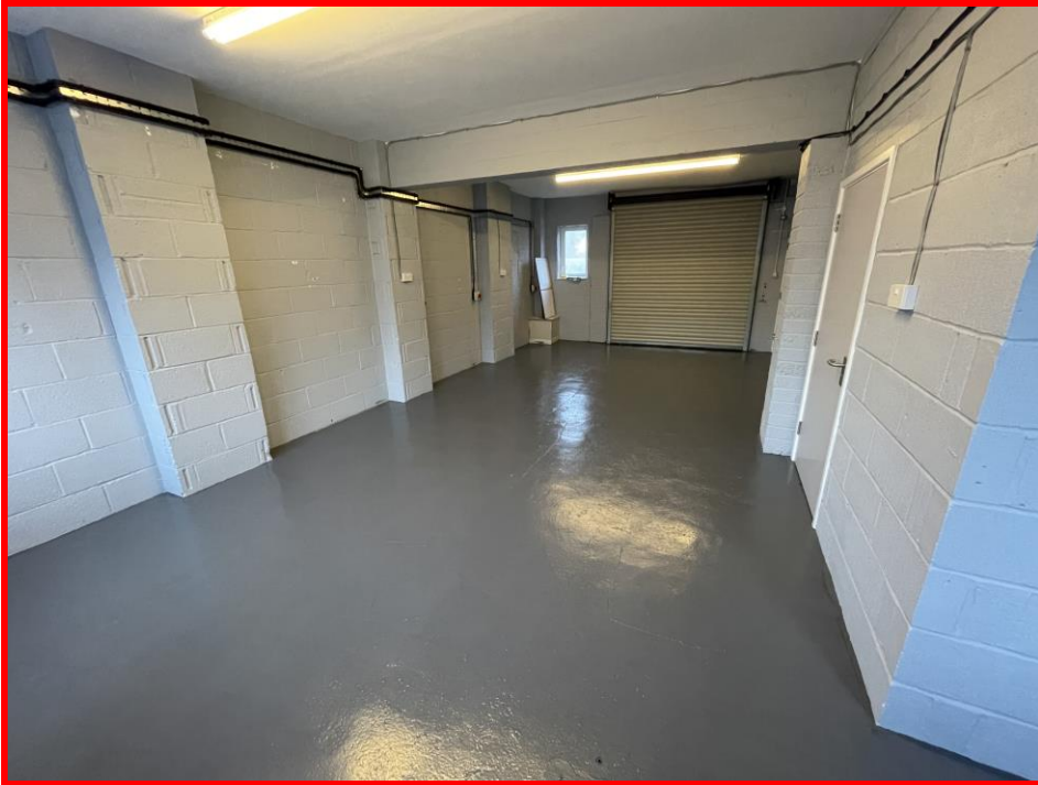
A ground floor historic interior picture showing unit 4 a similar unit within the estate
