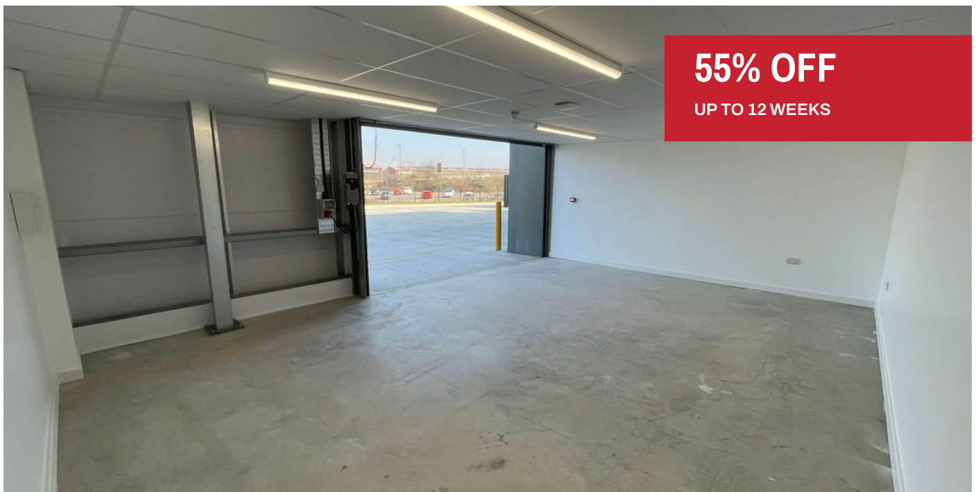
Ground-floor and drive-up units
